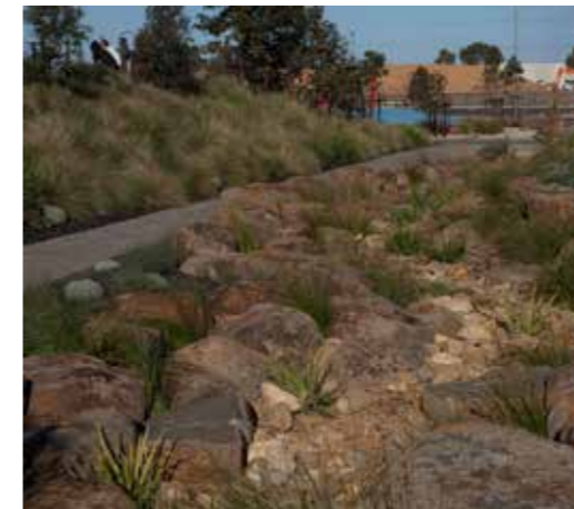
3 Rock stabilised embankment, revegetated where possible
