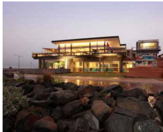
5 Use of timbers and glass
