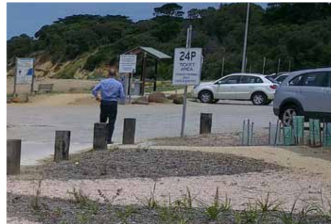
2 Permeable gravel parking areas
