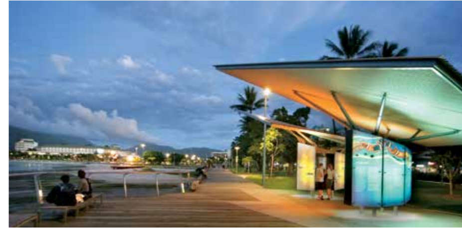
3 Interpretive shelter allowing for all weather access
