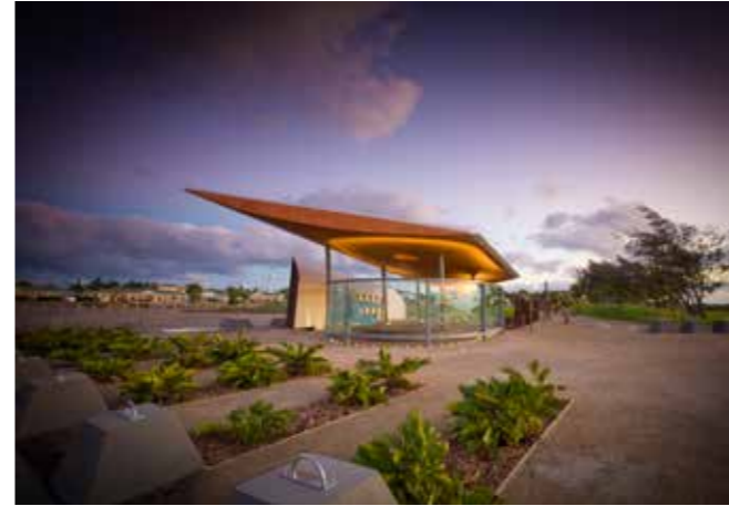
3 Gravel plaza space with low / ground cover planting to allow for views
