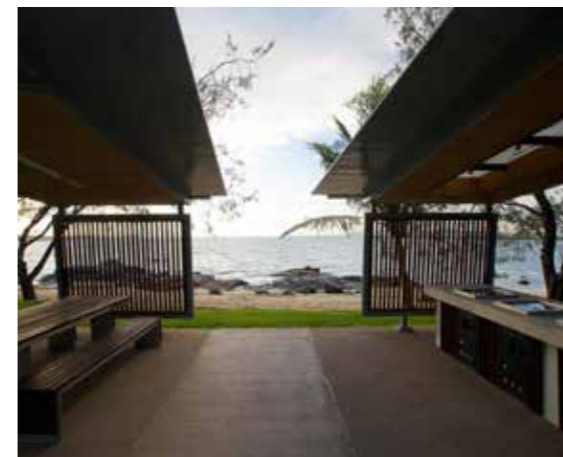
11 Built form framing views to water
