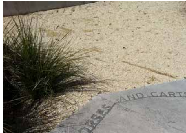
6 Gravel and uncoloured concrete
