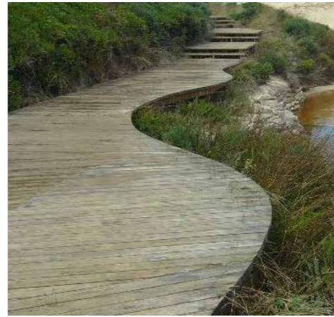
2 Timber board following form of embankment
