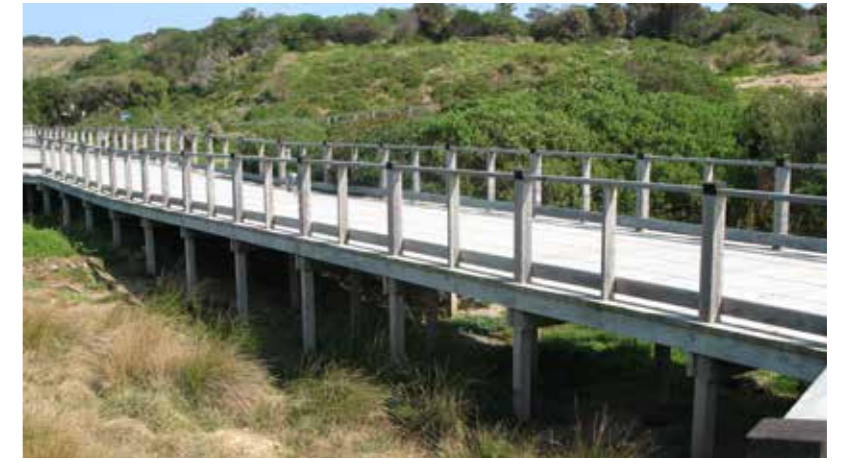
4 Timber board walk to navigate areas, where a path might not be appropriate
