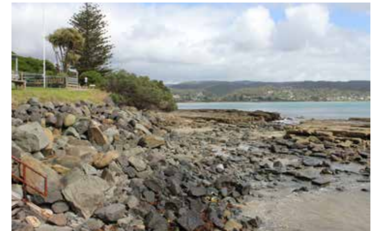
4 Existing foreshore edge (rock embankment)
