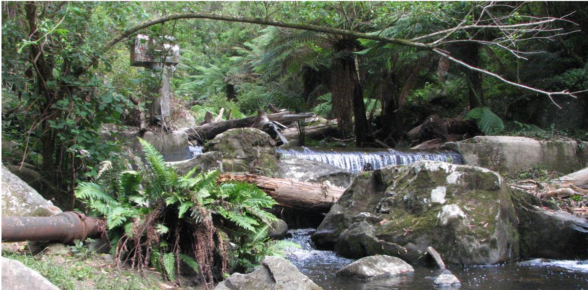
Figure 3. Remnants of past water supply system based on the Erskine River
