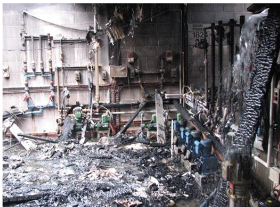
Figure 25 and 26 Damage to a water pumping plant which occurred during the 2009 Black Saturday fires
