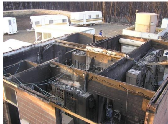
Figure 25 and 26 Damage to a water pumping plant which occurred during the 2009 Black Saturday fires
